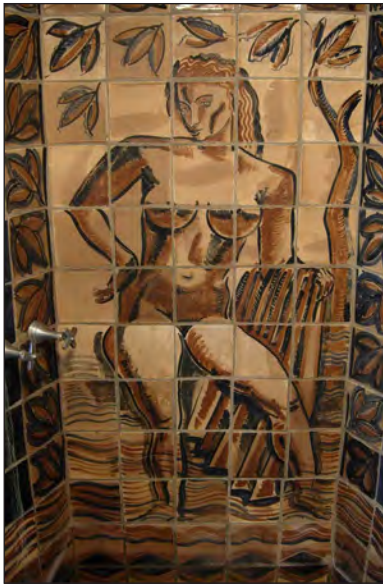
Shower tiles installed in Crow House in 1931.
