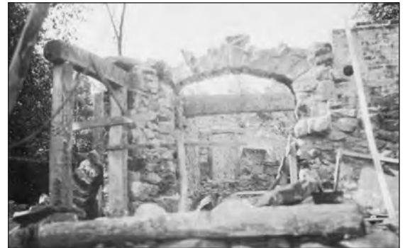
Crow House construction showing the archway from the kitchen into the living room
